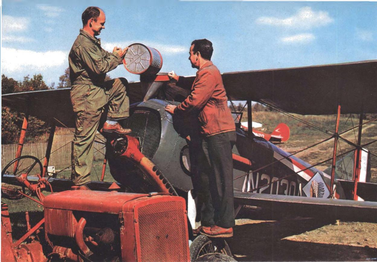
Water poured into radiator of the Spad's 180 hp Hispano-Suiza engine was later flung in Billman's face via leaks.
